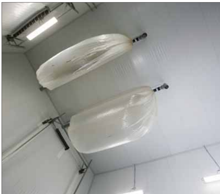
Buffer lungs regulate the atmosphere in the room partially before starting machinery.
