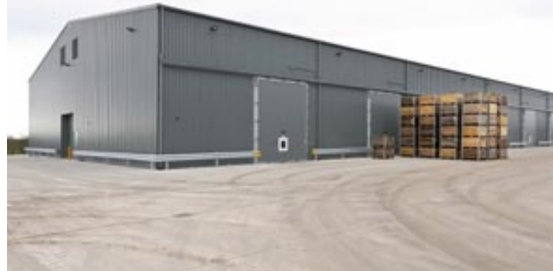
The newly constructed DCA fruit storage complex at AC Hulme & Sons' Hoaden Court.
